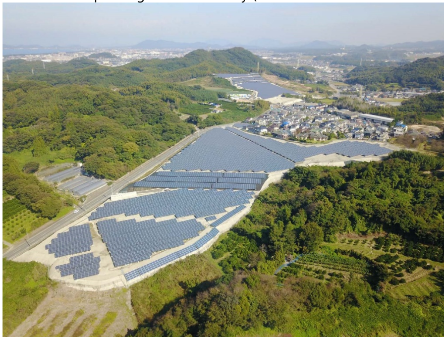
Panoramic view of power generation facility (one location in Fukuoka Prefecture)
