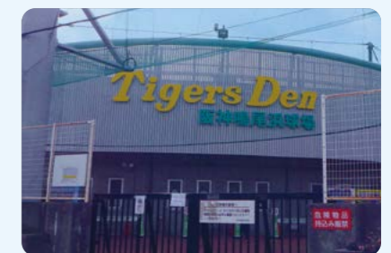
Hanshin Naruohama Baseball Stadium, where SMART undertook the demolition work
